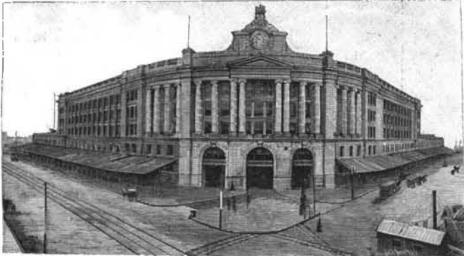
The Facade—Total Length of Station Front, 2,190 Feet.
