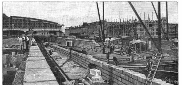
Subway for Suburban Tracks, and the Power Buildings.
