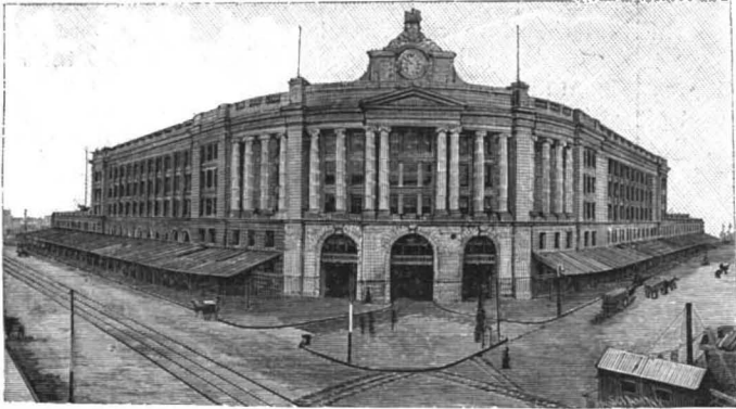
The Facade—Total Length of Station Front, 2,190 Feet.
