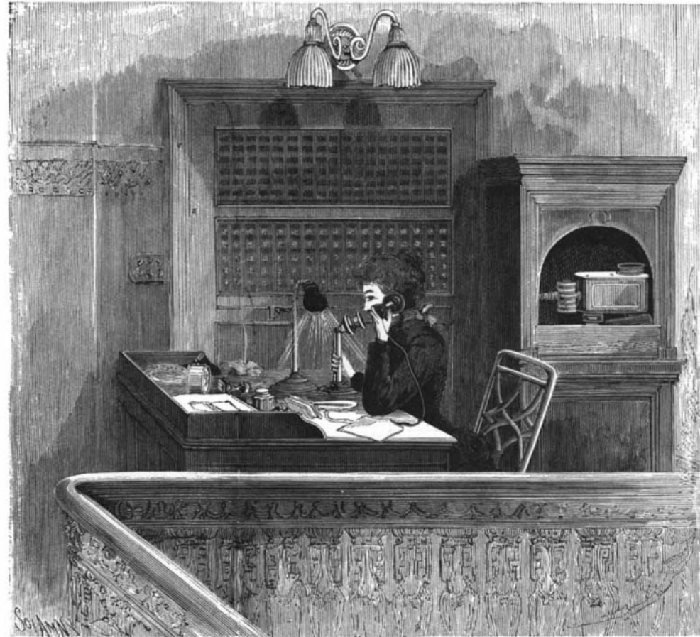
Local Floor Station.
