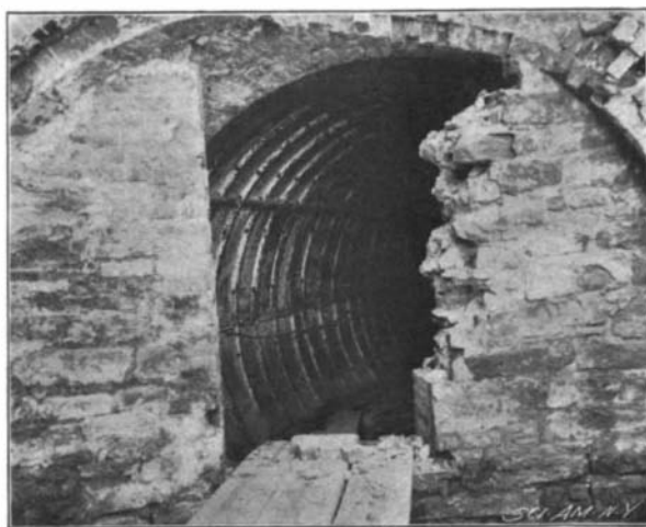
ENTRANCE TO THE BROADWAY TUNNEL.
