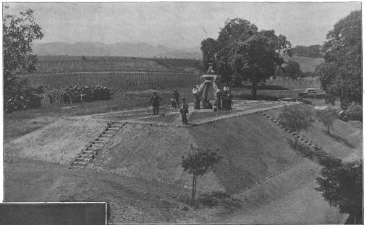
CEMENT TANK HOLDING 500,000 GALLONS.
