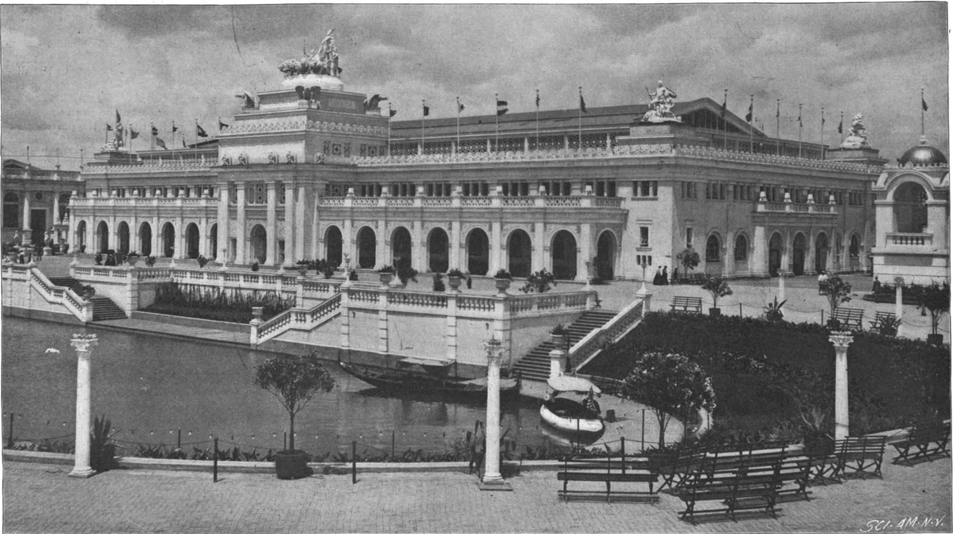
Machinery and Electricity Building.
