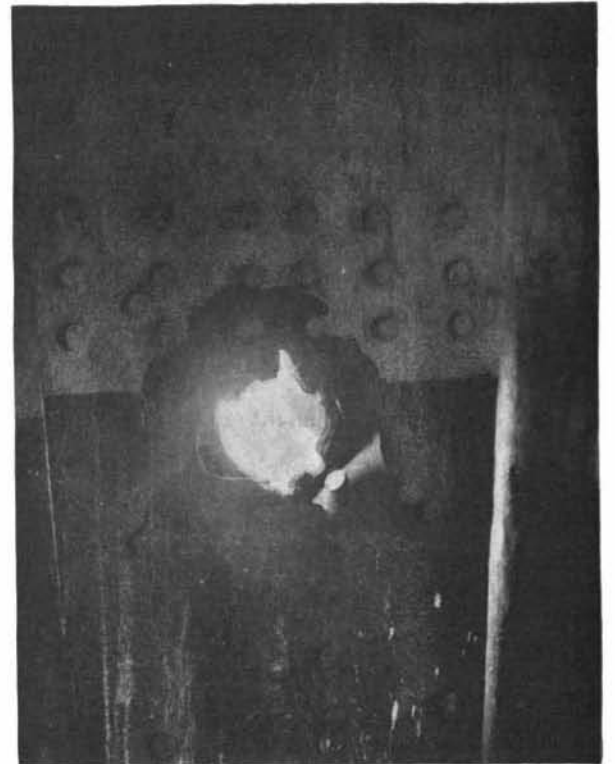
3.—Hole Made by 6-inch Shell in Port Bow on Gun Deck.
