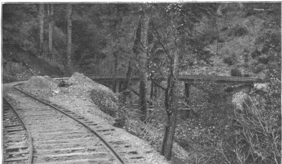
1.—A TYPICAL CURVE AND TRESTLE.
