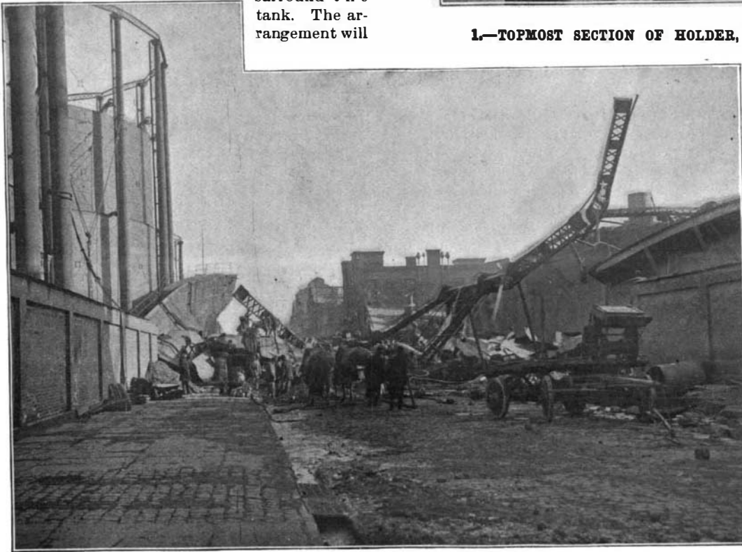
2.—WRECKAGE OF THE FRAME LYING ACROSS TWENTY-FIRST STREET.
