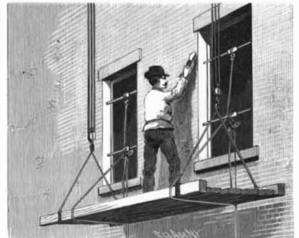
CODY'S SAFETY-ATTACHMENT FOR SCAFFOLDS.
