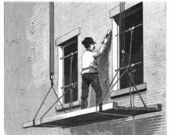
CODY'S SAFETY-ATTACHMENT FOR SCAFFOLDS.
