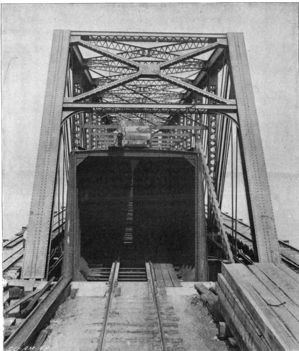
VICTORIA JUBILEE BRIDGE—END VIEW, SHOWING PIN-CONNECTED STRUCTURE ERECTED AROUND THE OLD TUBULAR BRIDGE.
