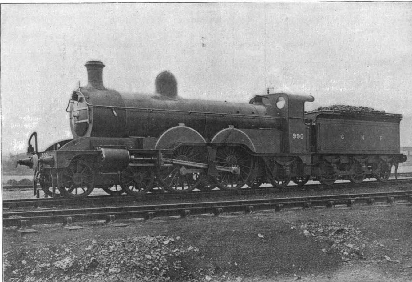
NEW TEN-WHEEL EXPRESS ENGINE FOR THE GREAT NORTHERN RAILWAY, ENGLAND.
