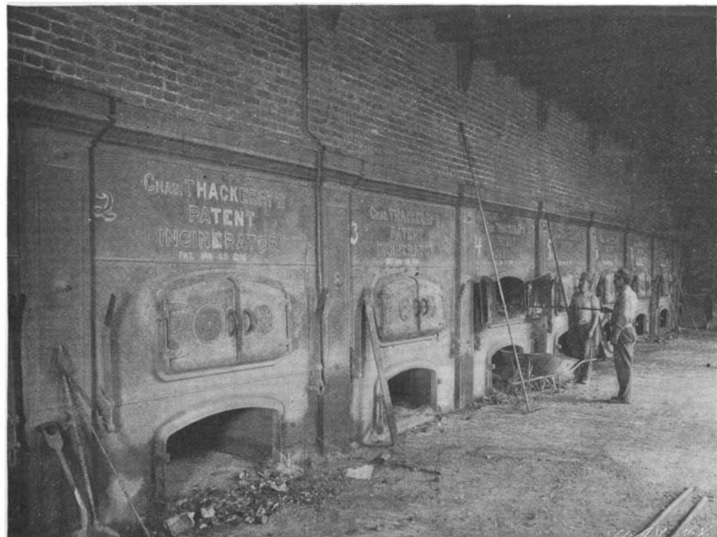
A SECTION OF THE INCINERATING FURNACE.
