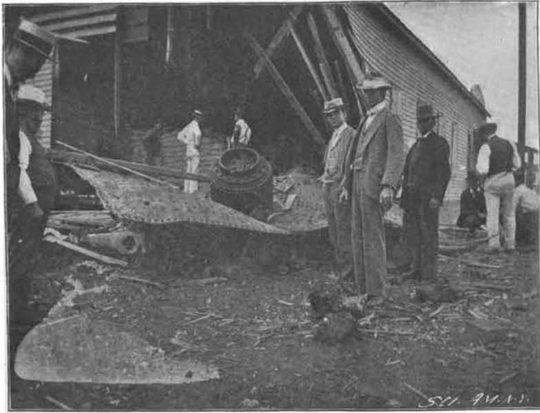
SHELL OF EXPLODED BOILER FOUND 1,200 FEET FROM ROUNDHOUSE.
