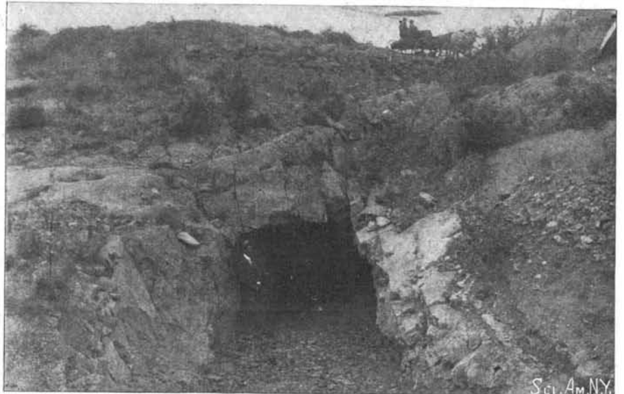
TUNNEL BENEATH A HIGHWAY.
