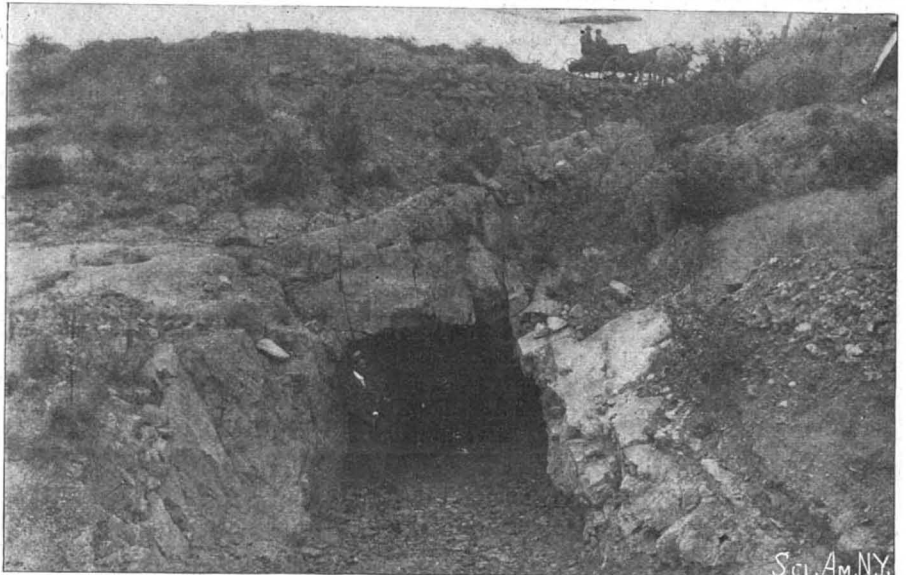
TUNNEL BENEATH A HIGHWAY.
