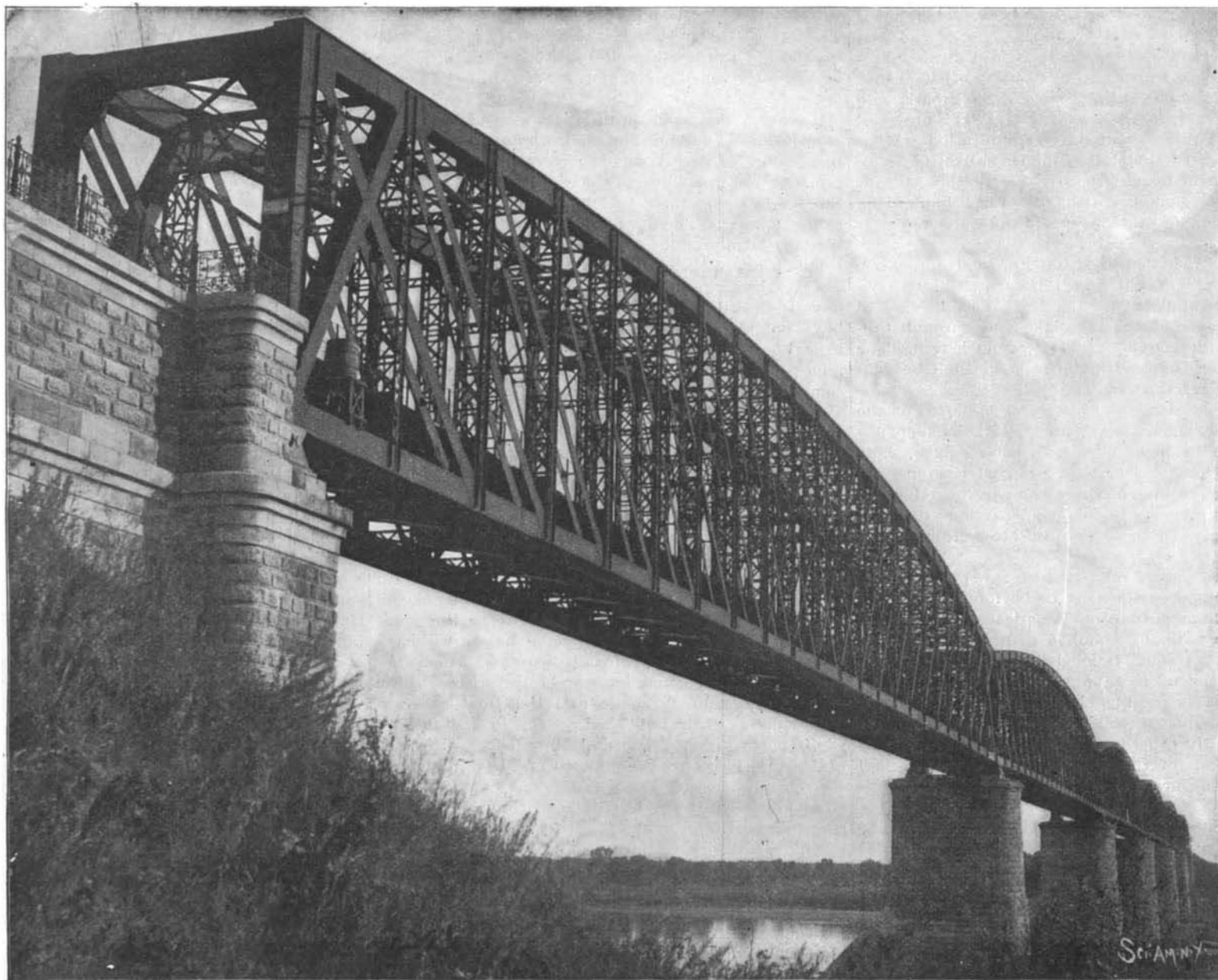
TRANSIBERIAN RAILWAY—STEEL BRIDGE AT OUFA, OVER THE BIELAIA RIVER.
