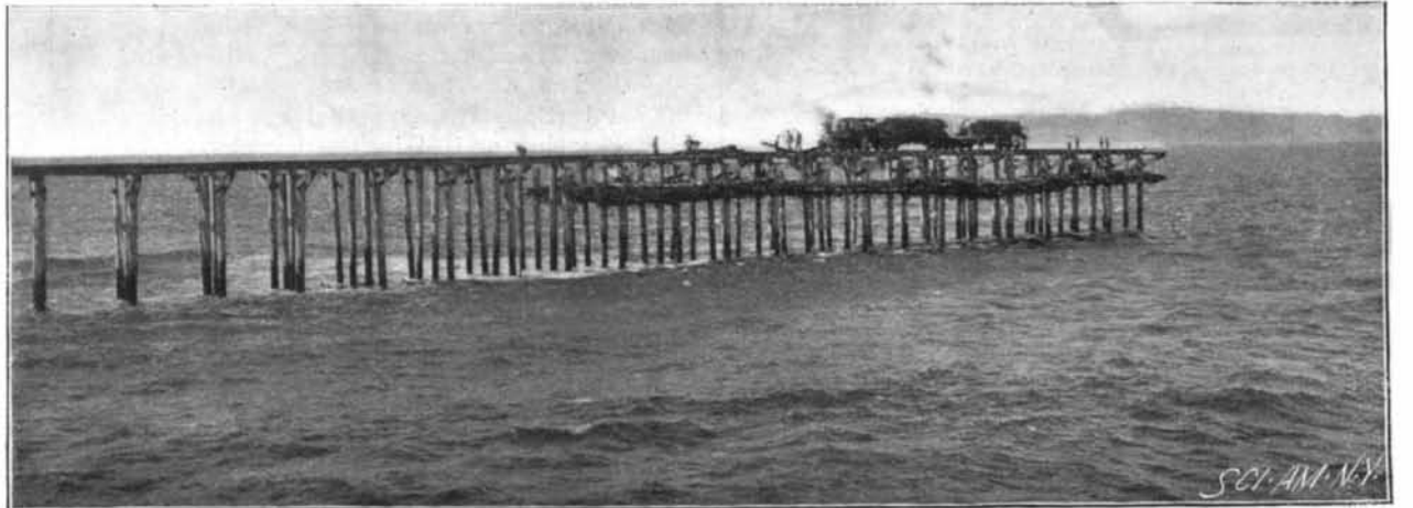
LOWERING AND LAUNCHING MATTRESSES AT SEAWARD END OF JETTY.
