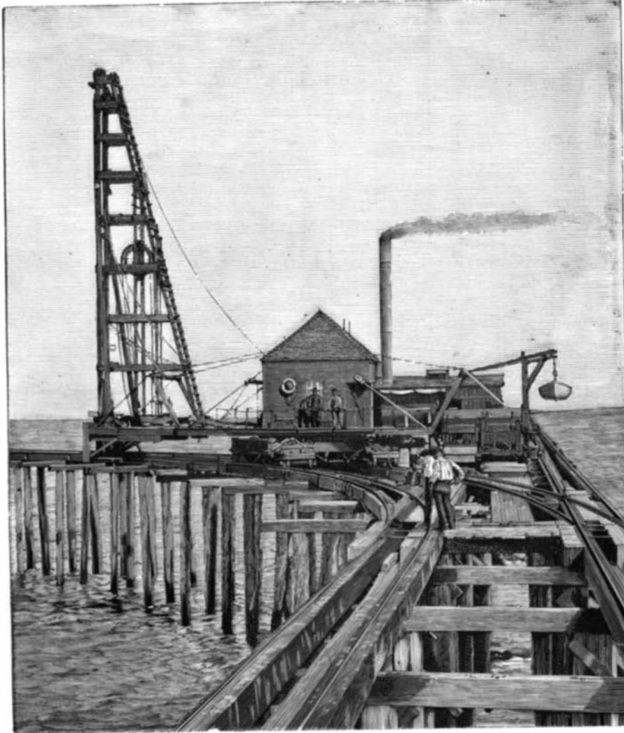
THE JET PILE-DRIVER USED IN CONSTRUCTING THE TRESTLE.
