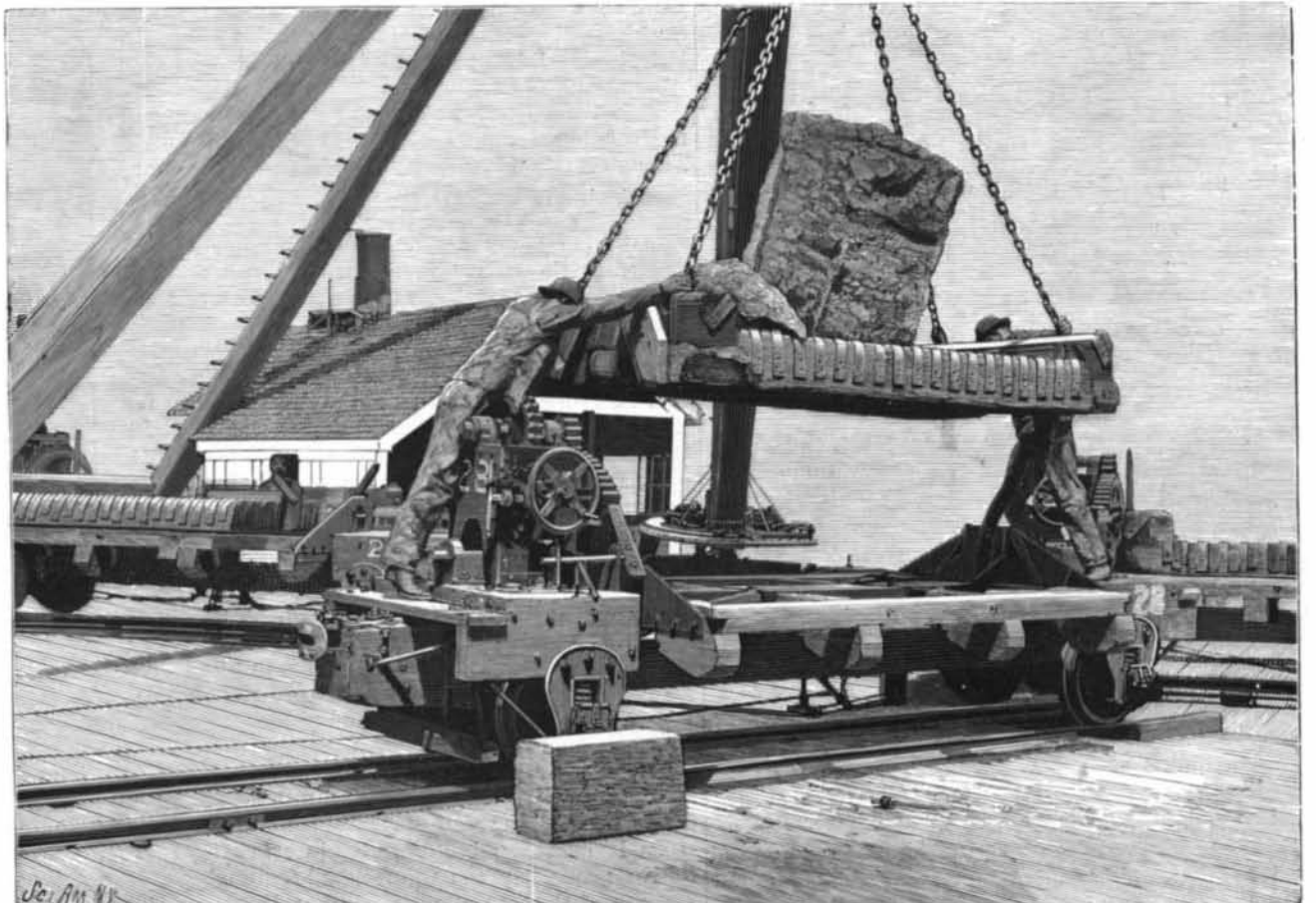
LOADING ROCK ONTO DUMP-CARS AT JETTY DOCK.
