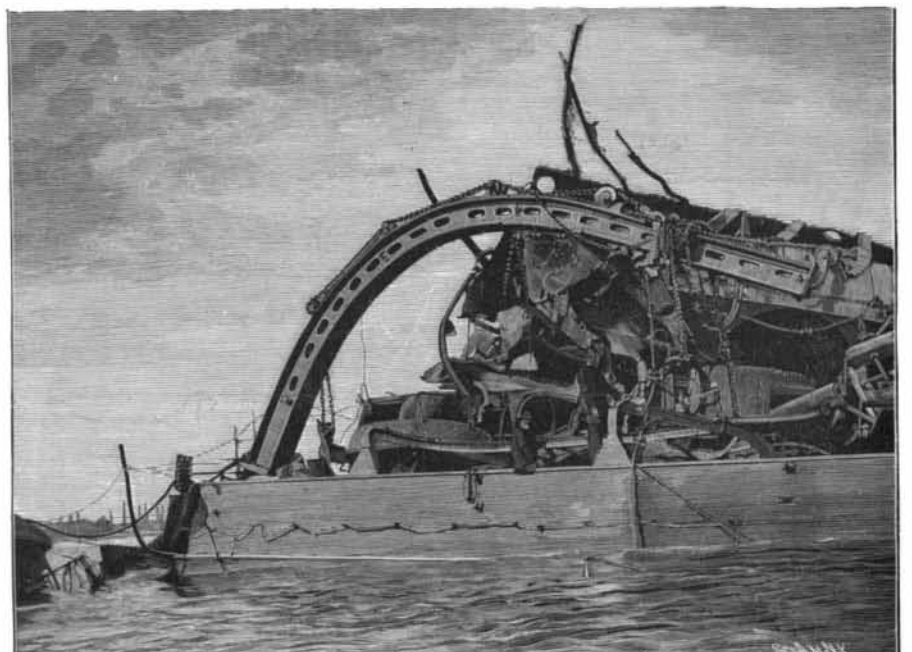
6.—THE FORWARD HALF OF SUPERSTRUCTURE DECK BLOWN OVER AND BACK UPON REAR HALF.
