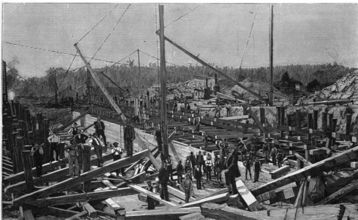
Fig. 3.—CONSTRUCTION OF LOCKS, DISMAL SWAMP CANAL.
