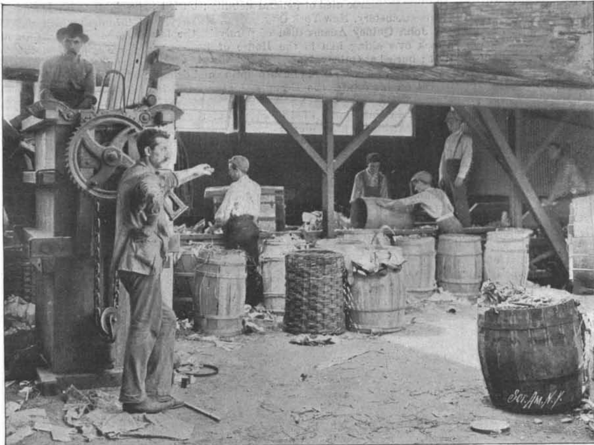
LOWER END OF SORTING TABLE NEAR THE FURNACE.
