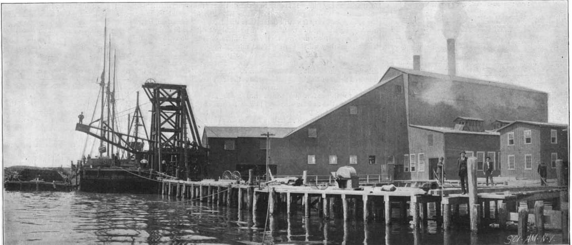
EXTERIOR OF GARBAGE WORKS.
