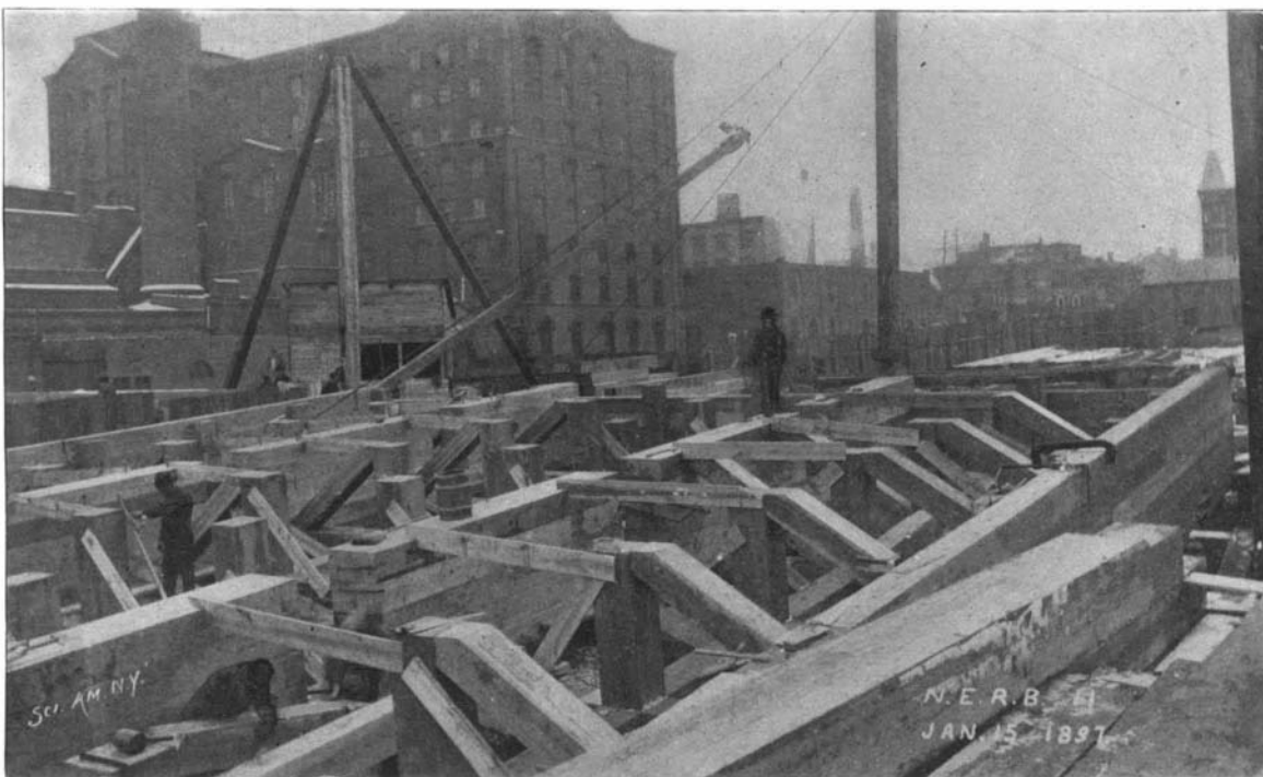
INTERIOR OF WORKING CHAMBER BEFORE ROOF IS BUILT ON.
