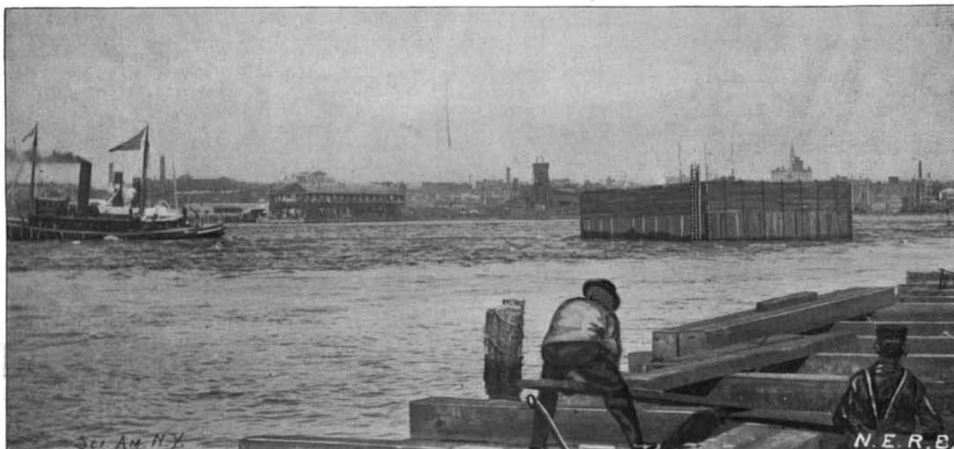
TOWING THE CAISSON TO SITE OF BRIDGE.
