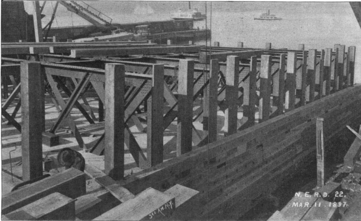
CONSTRUCTION OF CAISSON, SHOWING STEEL TRUSSES ABOVE THE ROOF.
