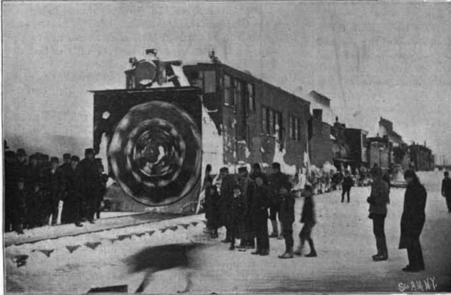
ROTARY PLOW PUSHED BY THREE ENGINES.
