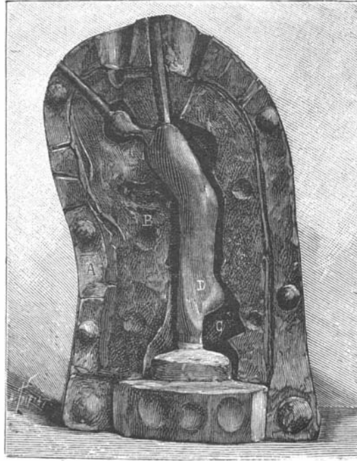
Fig. 2.—HALF MOULD, SHOWING THE DIFFERENT ELEMENTS.
