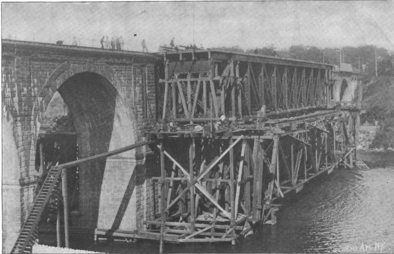
THE NEW STEEL SPAN READY FOR TRANSFERRING TO PLACE.
