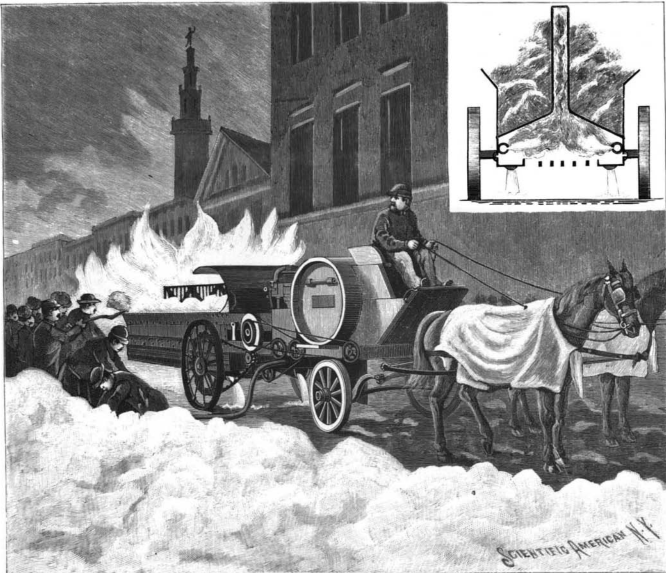
REMOVING SNOW FROM STREETS BY THE PROCESS OF MELTING.
