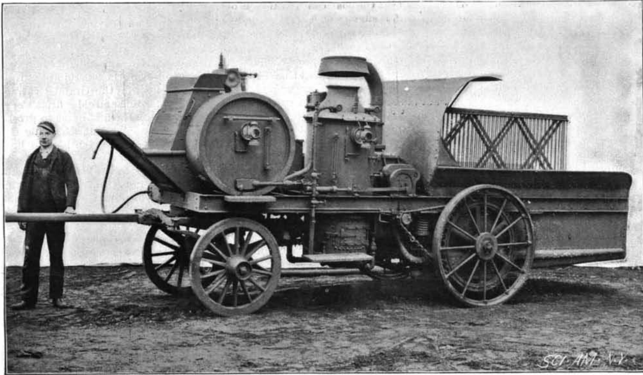
SNOW MELTING MACHINE NOW BEING USED IN THE STREETS OF NEW YORK.
