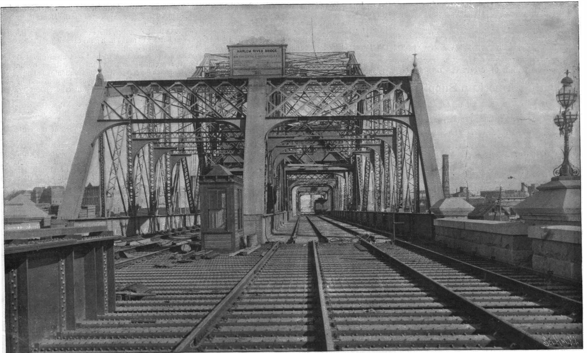
PORTAL VIEW OF THE FOUR TRACK STEEL DRAWBRIDGE.
