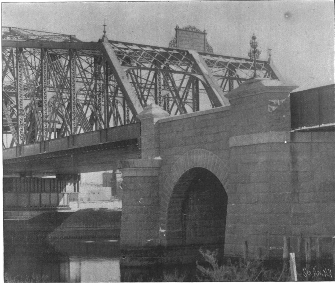
WEST ABUTMENT OF THE HARLEM RIVER BRIDGE.
