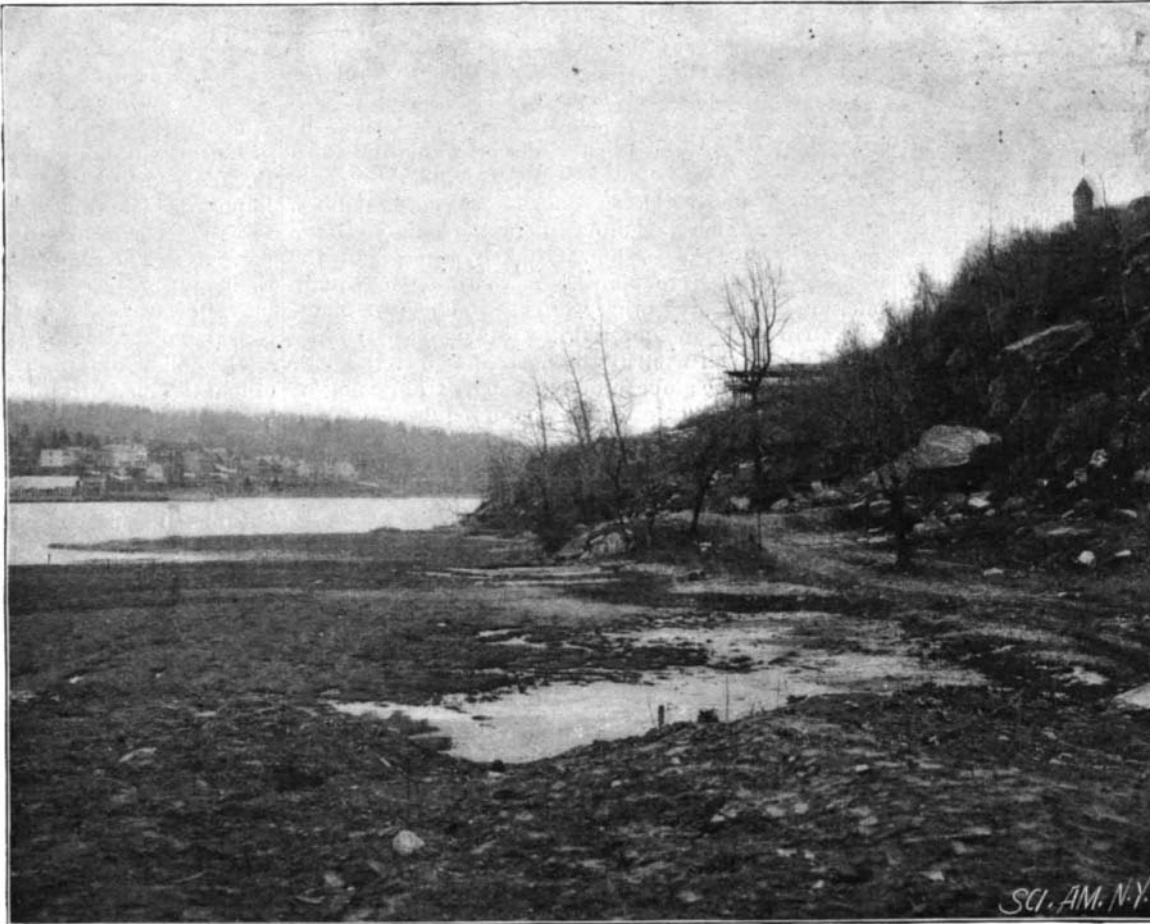
THE HARLEM RIVER SPEEDWAY—VIEW LOOKING SOUTH FROM DYCKMAN STREET BEFORE COMMENCEMENT OF WORK.
