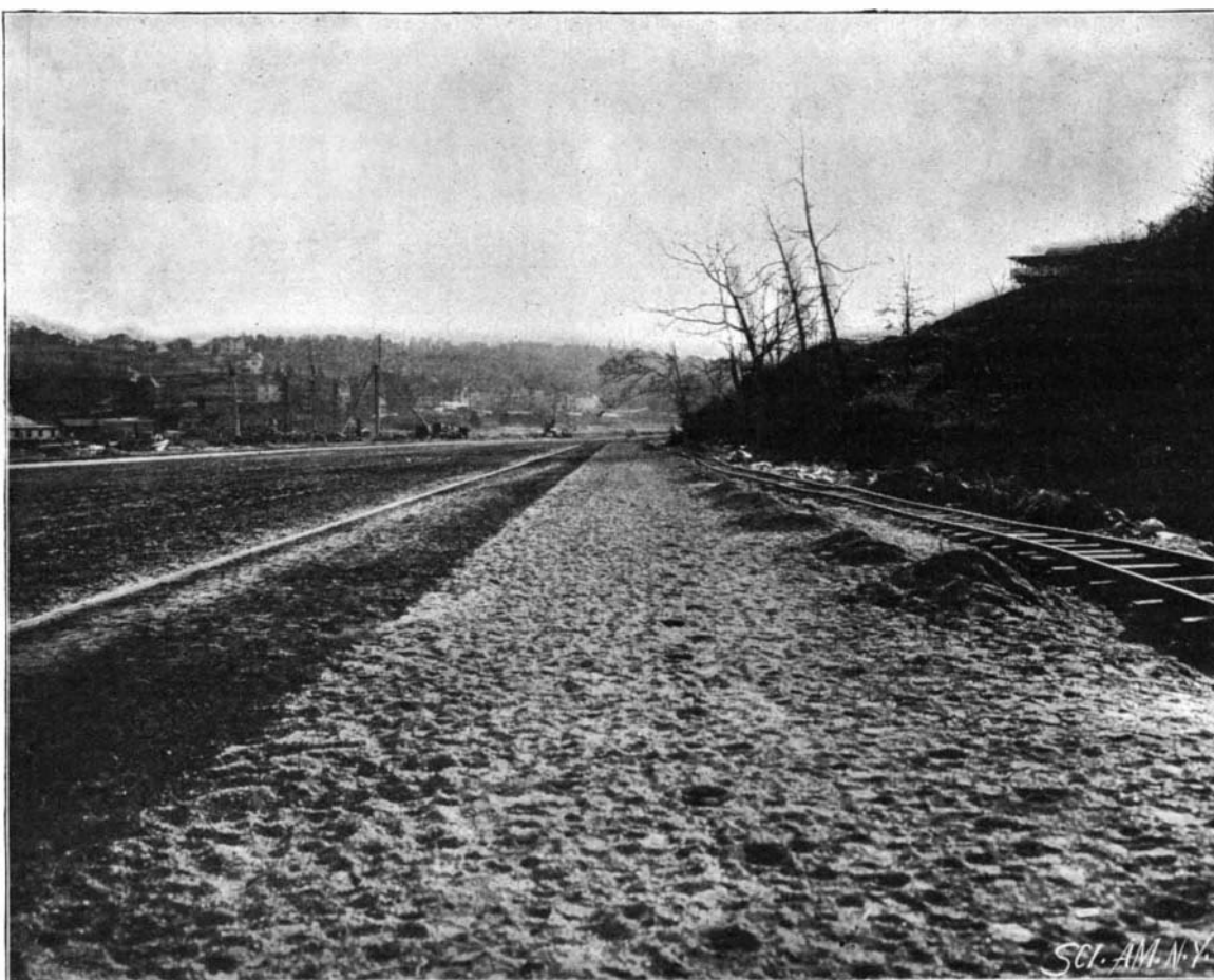
VIEW OF THE SAME SPOT SHOWING WORK COMPLETED.
