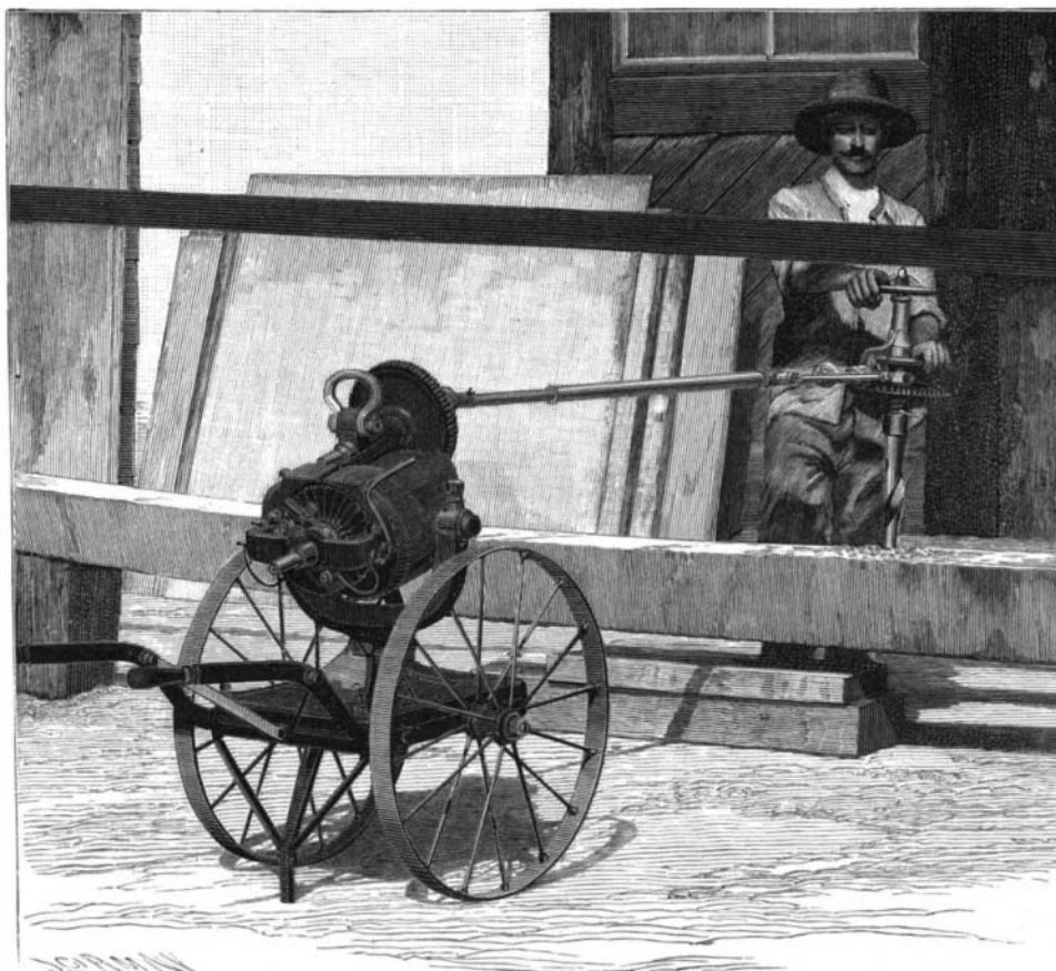
PORTABLE ELECTRIC DRILLING MACHINE AT WORK ON STEM OF LARGE STEAMSHIP.
