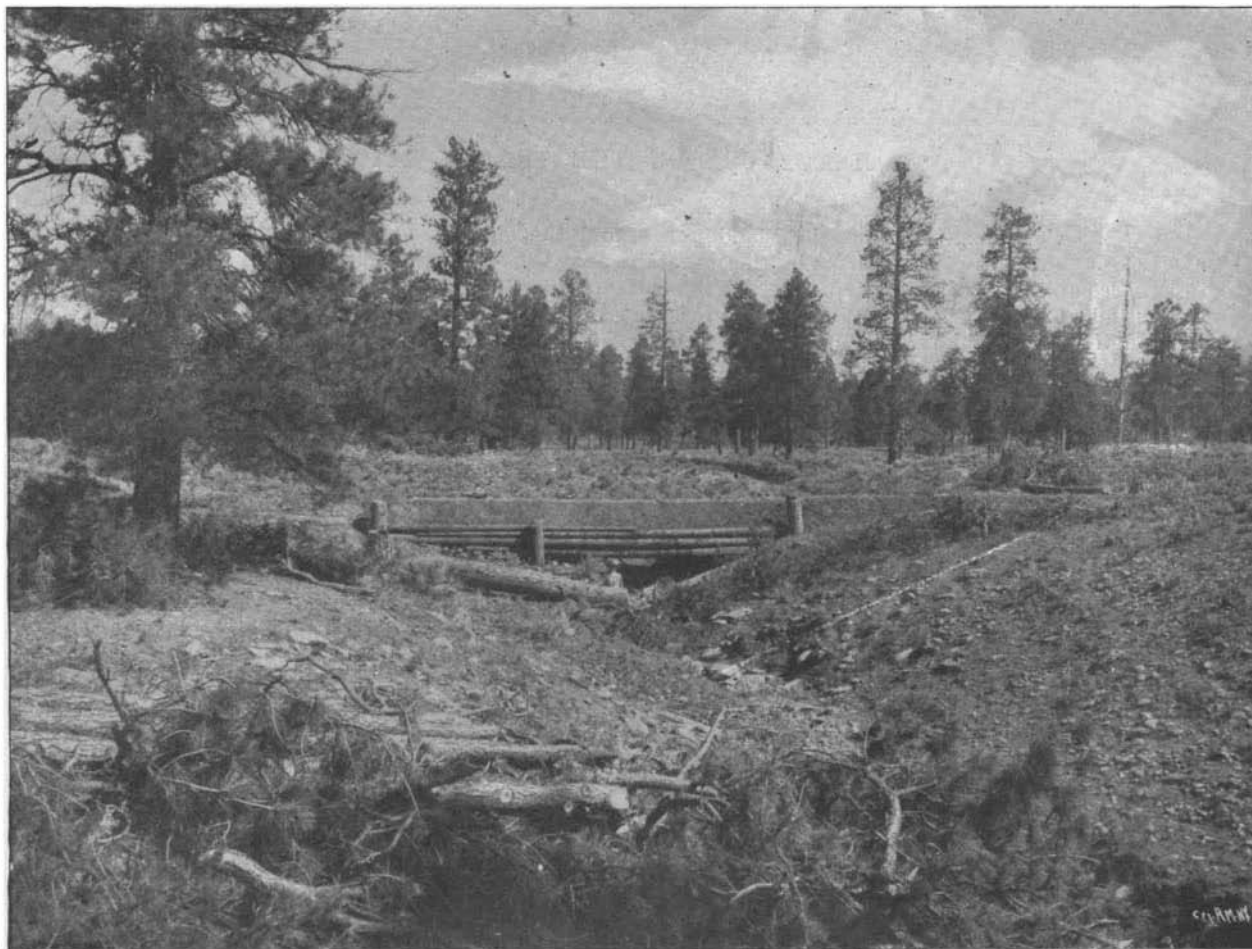
IRRIGATION NAVAHO RESERVATION—THE AQUEDUCT, WHEATFIELD DITCH.
