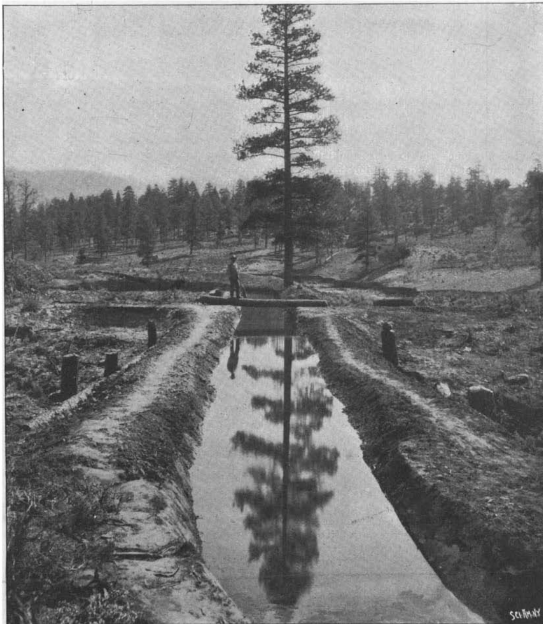
IRRIGATION WORK, NAVAHO RESERVATION.
