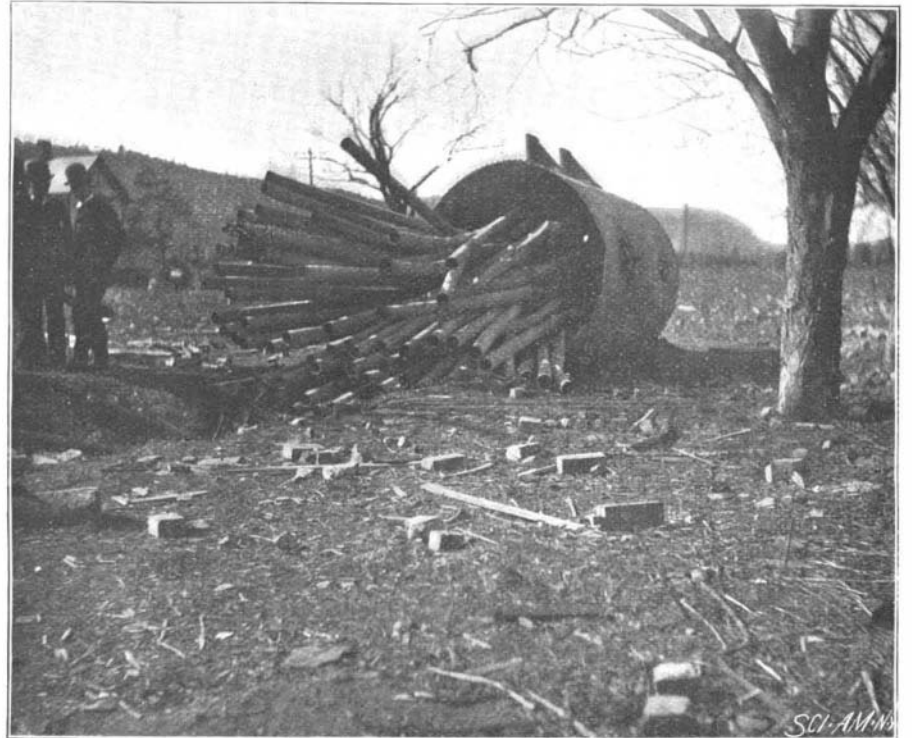
ONE-HALF OF BOILER IN FIELD 180 FEET DISTANT.
