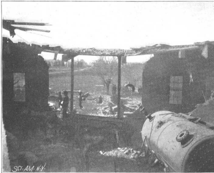
PATH CUT THROUGH BUILDING—PART OF BOILER 180 FEET DISTANT IN FIELD.
