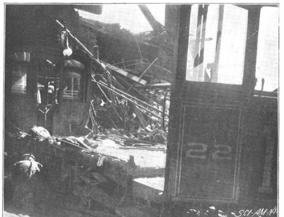
STREET CAR THROUGH WHICH PART OF BOILER PASSED.
