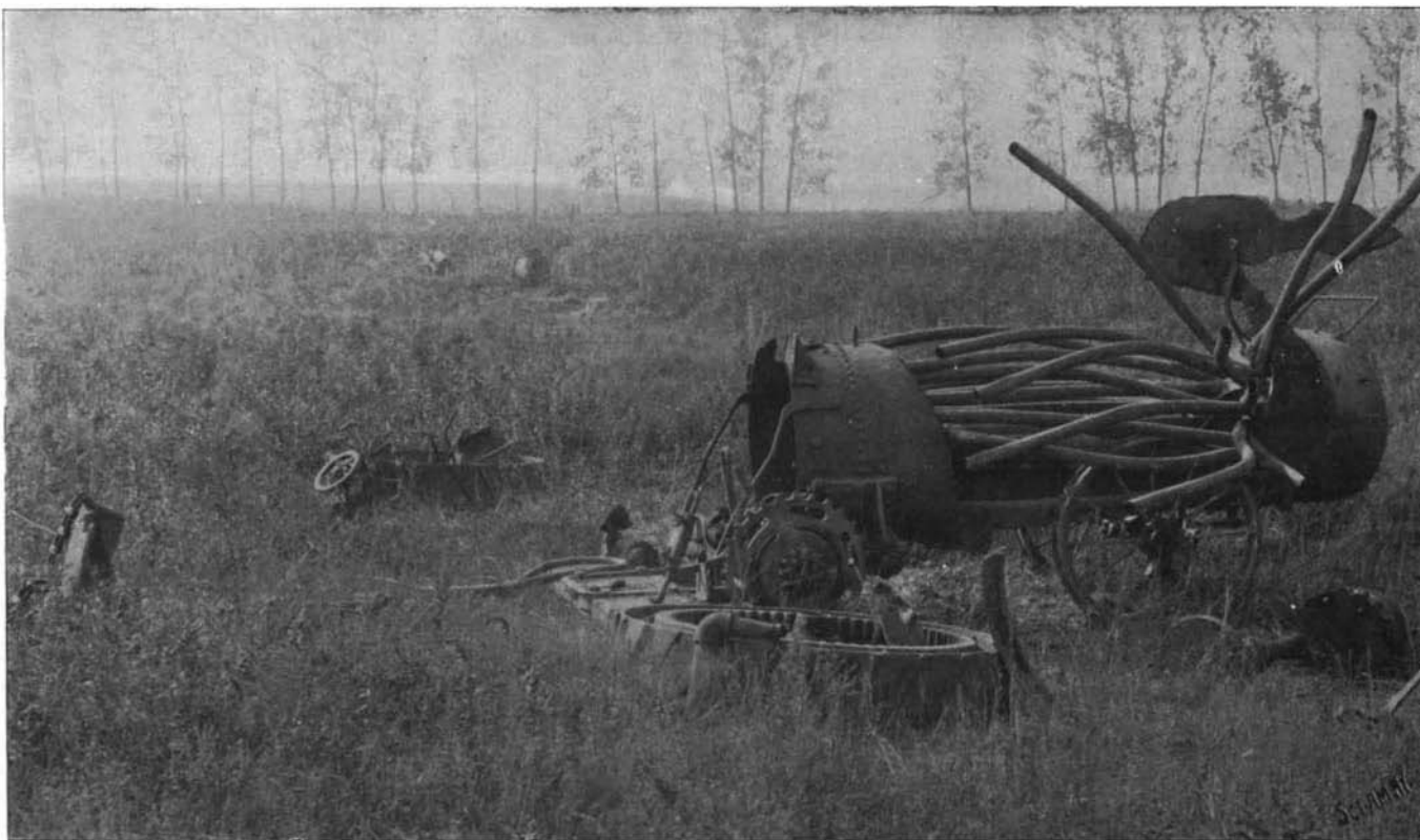
A TRACTION ENGINE BOILER EXPLOSION.
