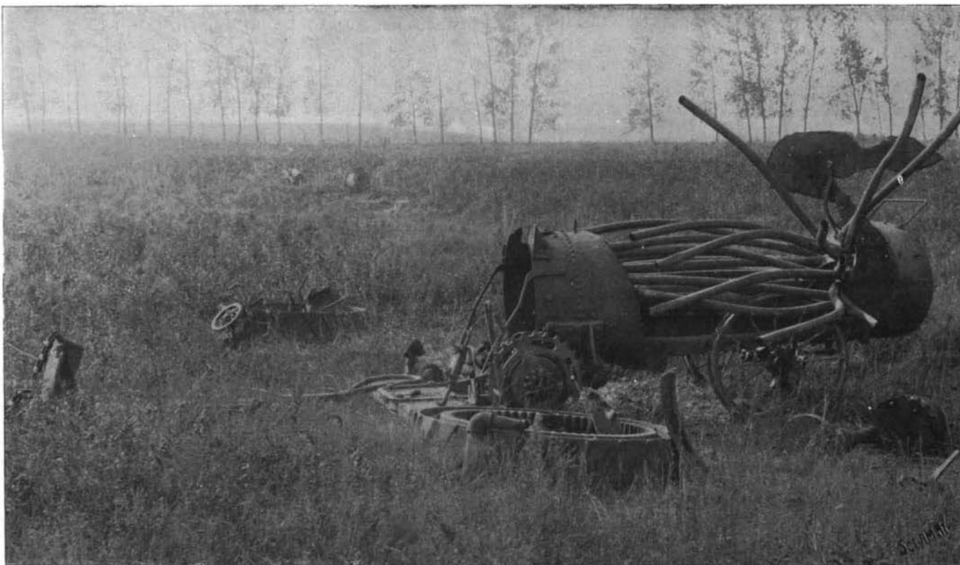
A TRACTION ENGINE BOILER EXPLOSION.
