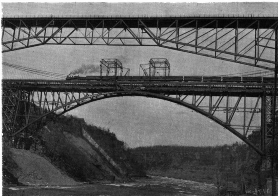
NEW STEEL ARCH BRIDGE OVER NIAGARA RIVER.
