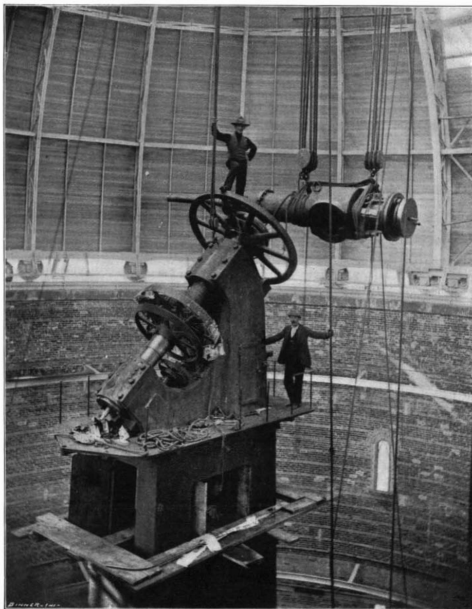
ERECTING THE DECLINATION AXIS OF THE YERKES TELESCOPE.
