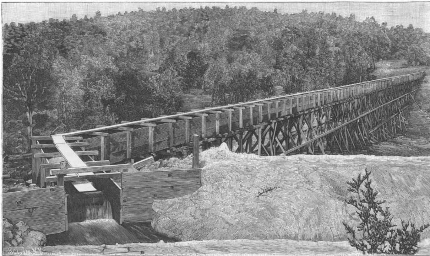
Fig. 9.—DIVERSION FLUME FOR BRINGING WATER TO THE RESERVOIR.
