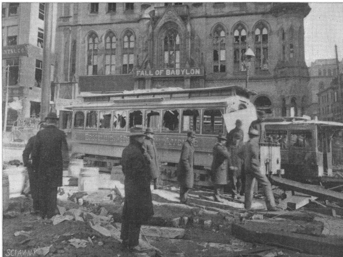
CARS WRECKED BY THE BOSTON GAS EXPLOSION.
