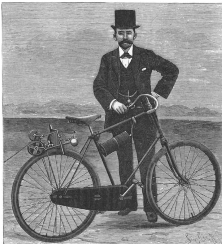
TELEGRAPH LAYING CYCLE.
