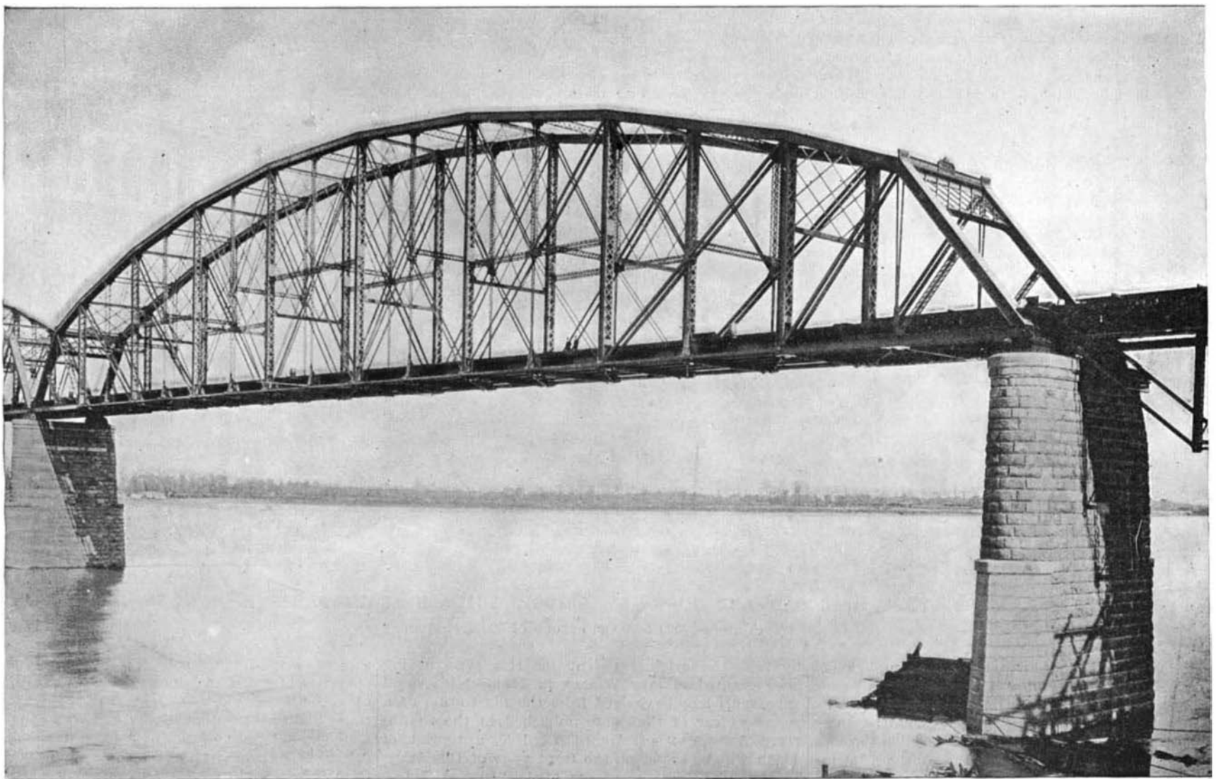
THE MERCHANTS' BRIDGE, ST. LOUIS—TYPICAL MODERN DOUBLE TRACK STEEL RAILROAD BRIDGE. Three spans, 517 feet 6 inches, and six spans, 125 feet long.
