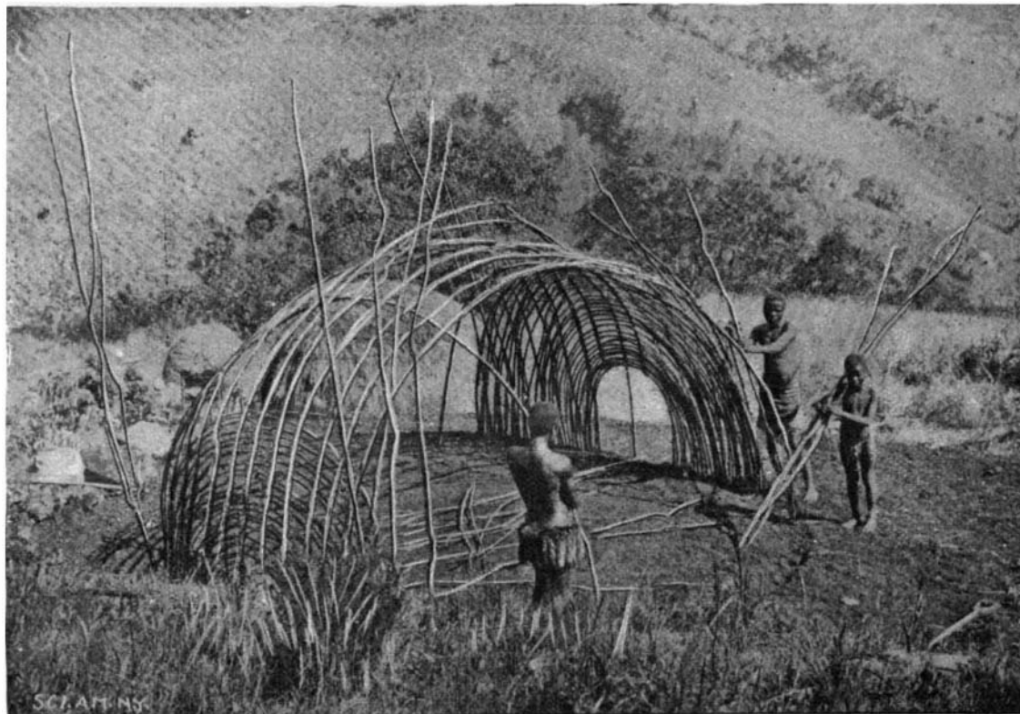
A HUT IN PROCESS OF CONSTRUCTION.
