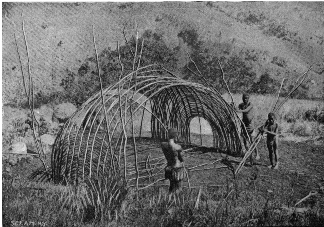
A HUT IN PROCESS OF CONSTRUCTION.
