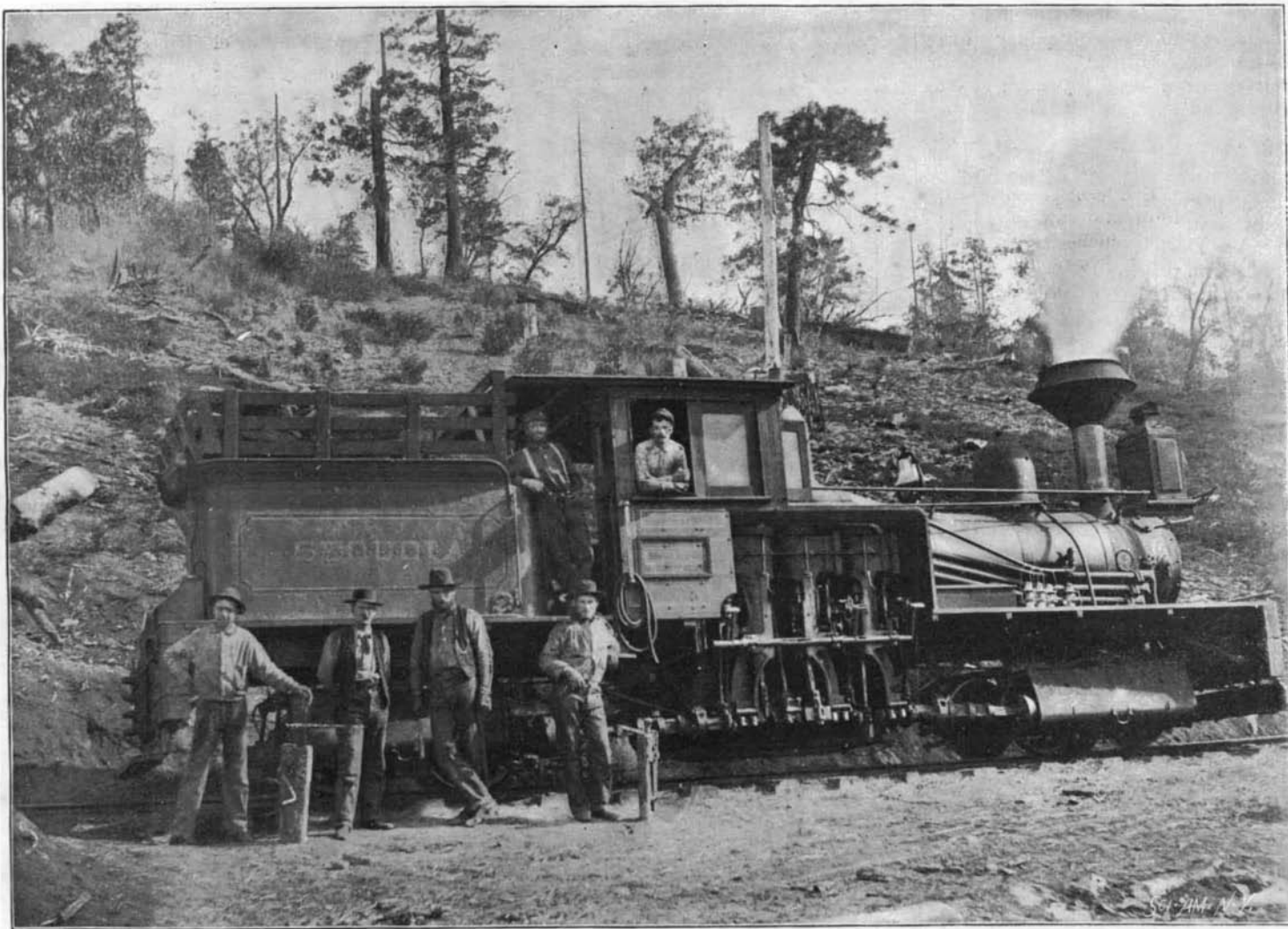
LOGGING IN THE SIERRA NEVADAS—A THREE CYLINDERED MOUNTAIN LOCOMOTIVE.
