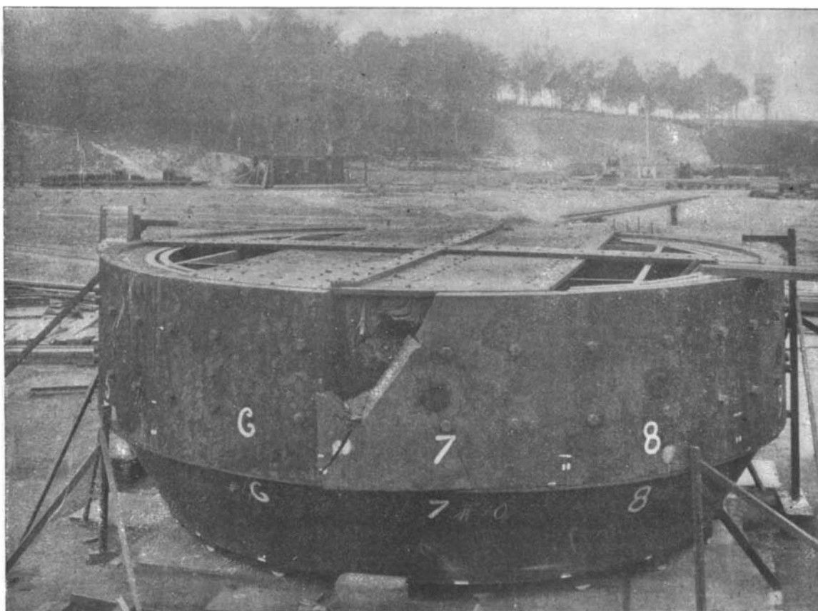
EXTERNAL VIEW OF REAR WALL, SHOWING DESTRUCTION OF 15 INCH PLATE BY FRAGMENT OF SHOT WHICH PASSED THROUGH TURRET. 12 INCH GUN SHOWN IN THE DISTANCE.
