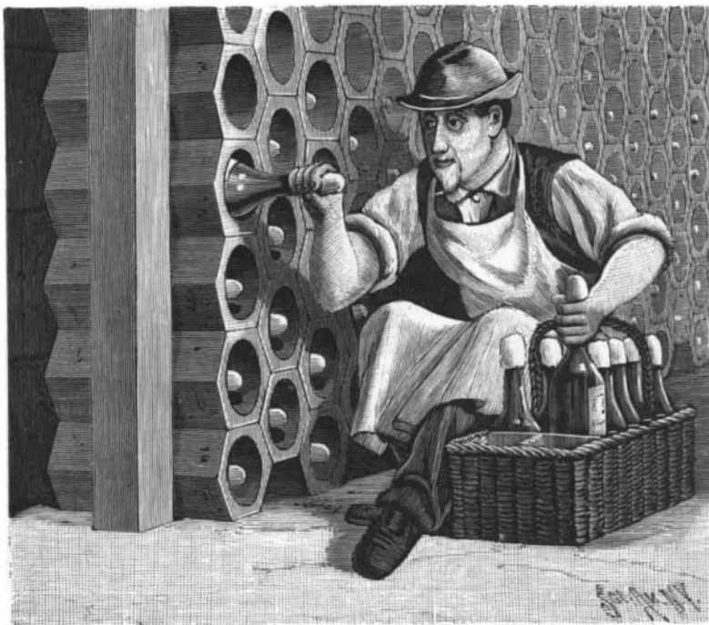
HONEYCOMB WINE BINS OF VITRIFIED CLAY PIPE.
