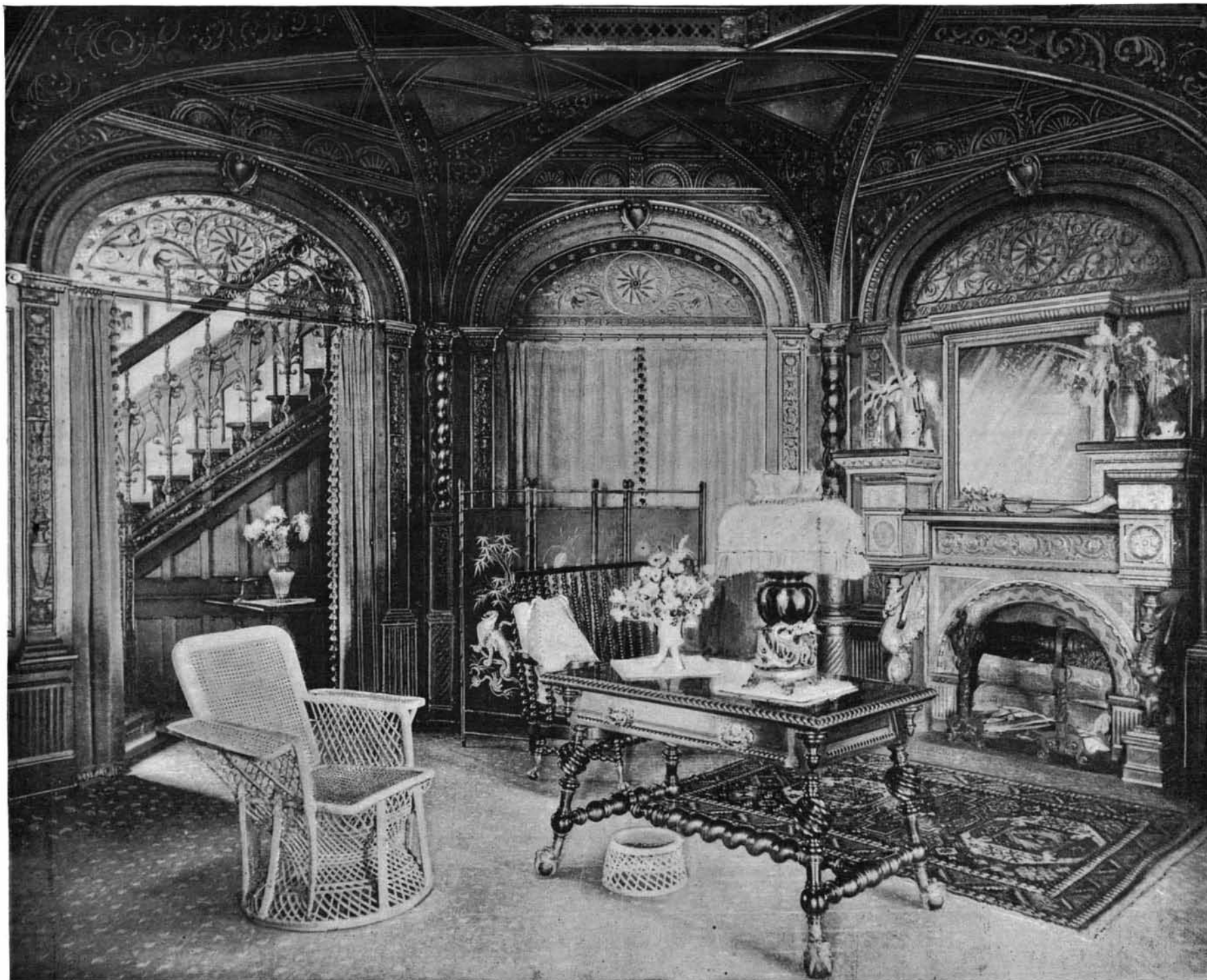
IRON AND COPPER IN HOUSE CONSTRUCTION AND DECORATION—MAIN HALL, SHOWING METAL CEILING AND WAINSCOTING.
