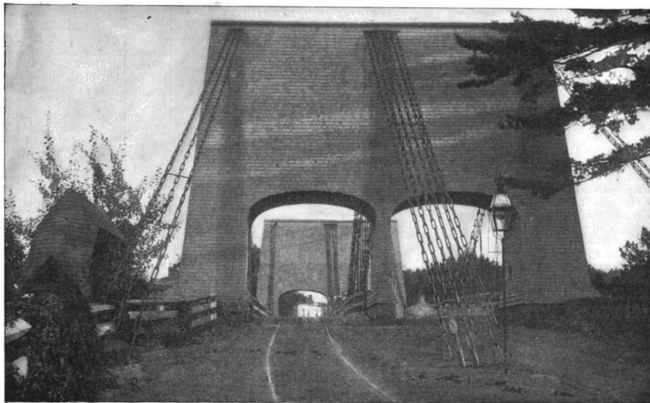
ANCHORAGE OF ESSEX-MERRIMAC CHAIN SUSPENSION BRIDGE.
