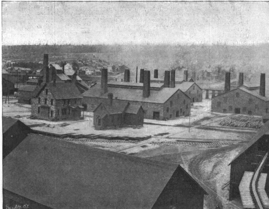
CALUMET AND HECLA SMELTING WORKS.
